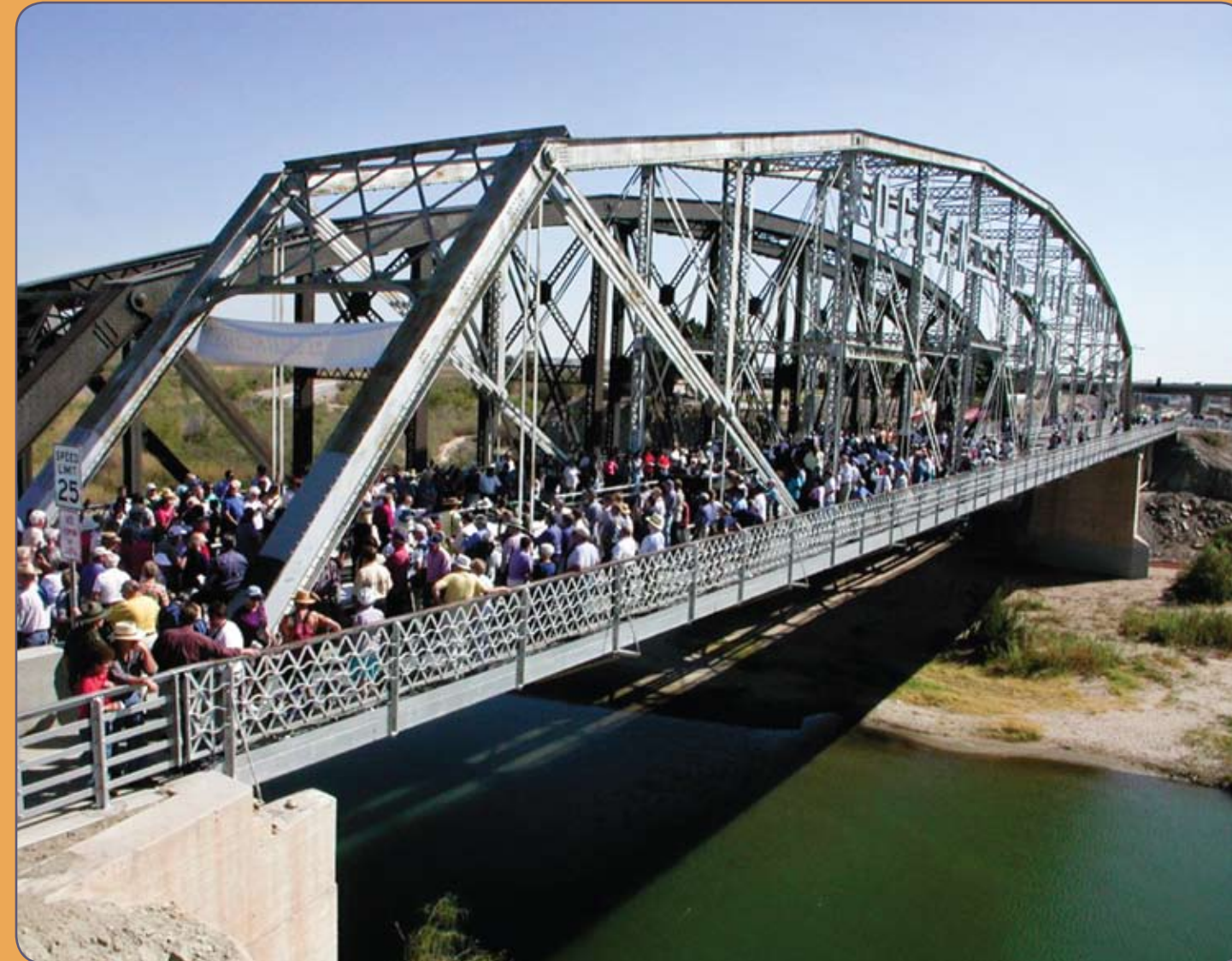
February 28, 2002, was a pivotal day in the life of the Yuma community: The reopening of the Ocean-to-Ocean Bridge. The Quechan Indian Tribe and the City of Yuma worked together to make this happen, and helped build a partnership which made restoration of the East Wetlands a reality.
