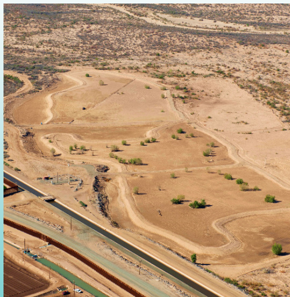
Right: Photo of Hunters Hole Conservation Area prior to construction.
