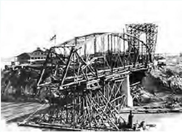
Building the Ocean-to-Ocean Bridge—1915
