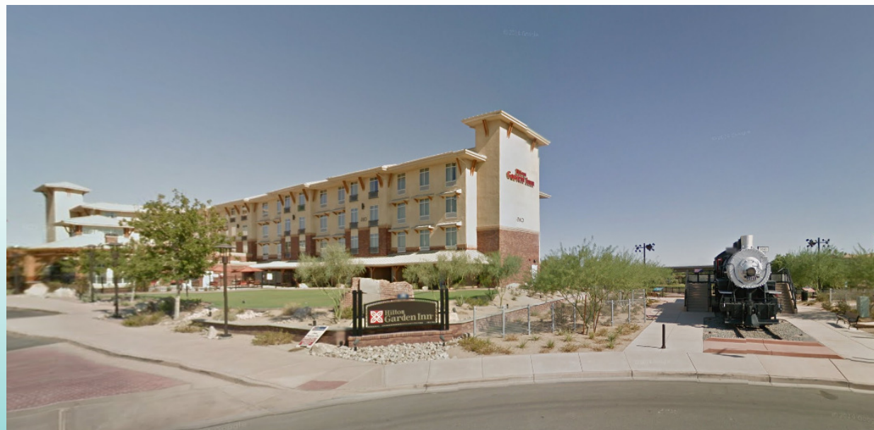
Below: Hilton Garden Inn and Conference Center in 2011- Construction of the site after the Settling Tanks were removed.
